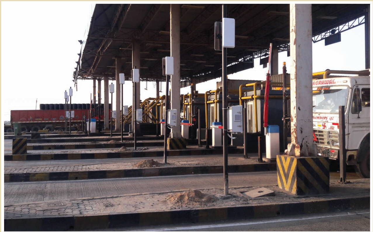
RFID Readers installed at Mokha Toll Plaza, Gujarat under DMICDC's Logistics Data Services Project
