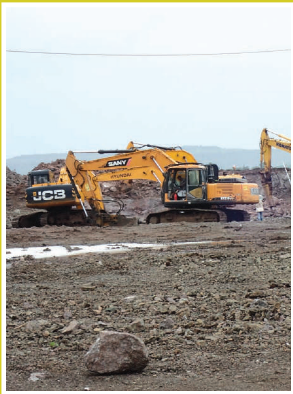
Site Leveling works being undertaken by HYOSUNG
