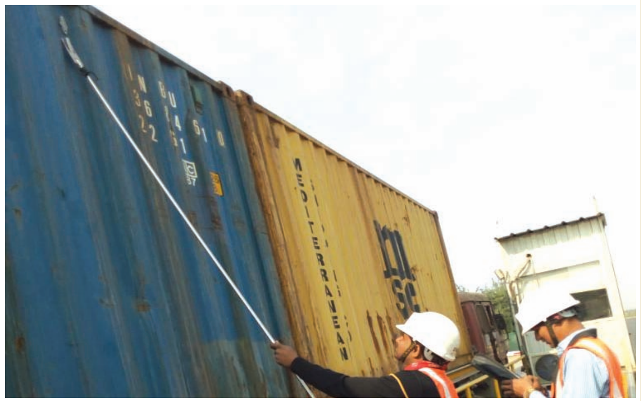
RFID Tagging of Containers at Ports under DMICDC's Logistics Data Services Project
